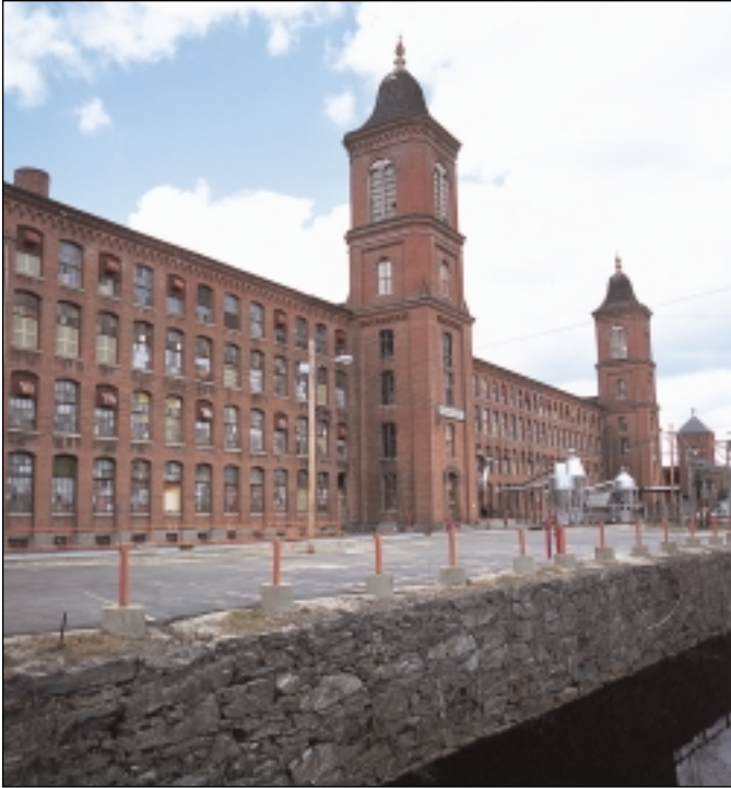
FIGURE 1.19 Industrialization in the 1800s. A textile mill in North Grovnerdale, Connecticut. Built in 1872 beside a canal, its four floors enabled steam power based on burning coal to be used more efficiently.
