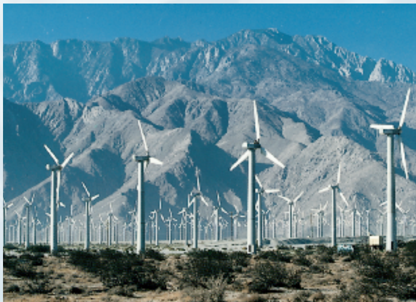
Figure 3-42 Wind turbine “farm” near Palm Springs, California. Such farms consist of as many as several hundred turbines and can supply energy to tens of thousands of homes and businesses. About 1 percent of the electricity used in the United States in 2003 had wind as its source.
