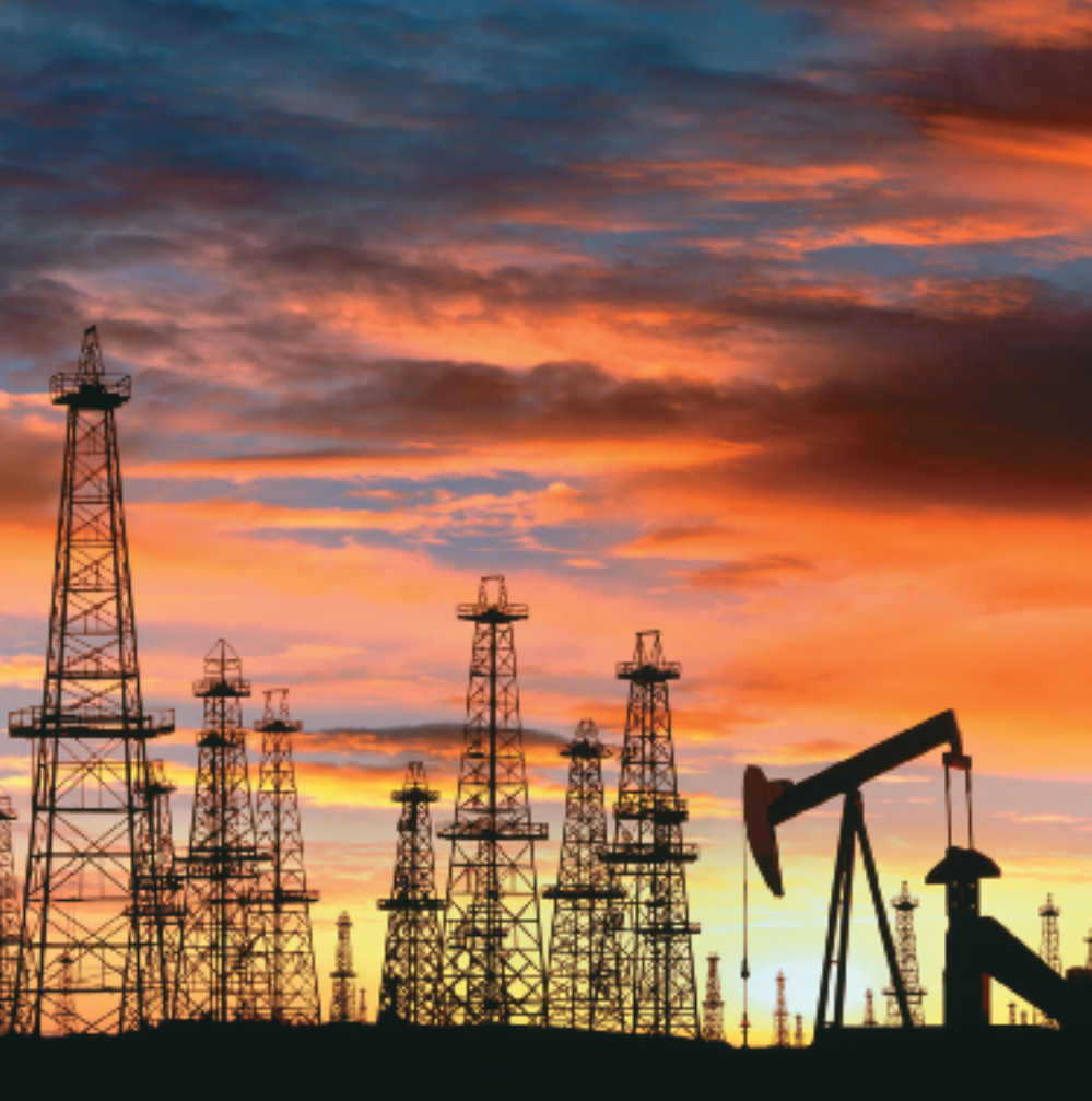
Oil wells in California.
