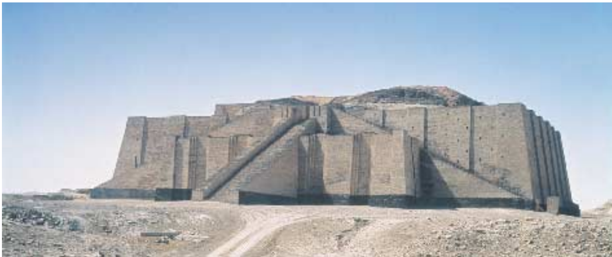
Figure 1.9 Ziggurat of Ur. Ca. 2100 B.C. Ur (Muqaiyir, Iraq). A temple to Nanna, the moon god, stood on the top of the ziggurat, which was terraced on three levels. On the first level was an entranceway approached by two sets of steps on each side and one in the front. The base, or lowest stage, which is all that remains of this “Hill of Heaven,” measures 200 by 150 feet and stands 70 feet high. In comparison, Chartres cathedral in France is 157 feet wide, with each tower over 240 feet high.
