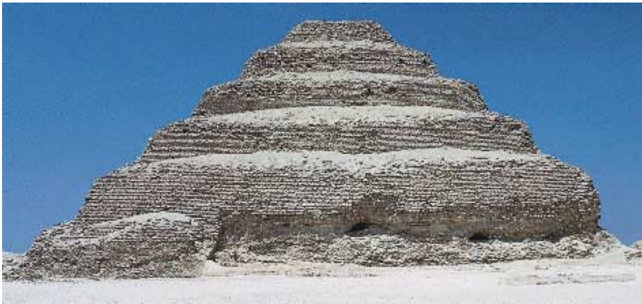
Figure 1.12 IMHOTEP. Step Pyramid of King Djoser. Ca. 2680 B.C. Sakkareh, Egypt. Though isolated from its neighbors until about 1730 B.C., Egypt was influenced by surrounding cultures, as the design for the step pyramid at Sakkareh shows. Resting on a rectangular base and rising in six progressively smaller stages, this pyramid was modeled on Mesopotamia's ziggurat. But unlike the ziggurats, which were made of dried clay bricks, it was built of cut stone, the first building to be so constructed in the world. The step pyramid has six levels on a 411- by 358-foot base and stands 204 feet high.
