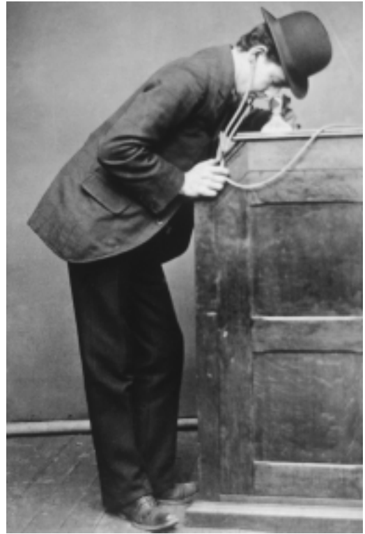
Courtesy of the Edison National Historic Site
