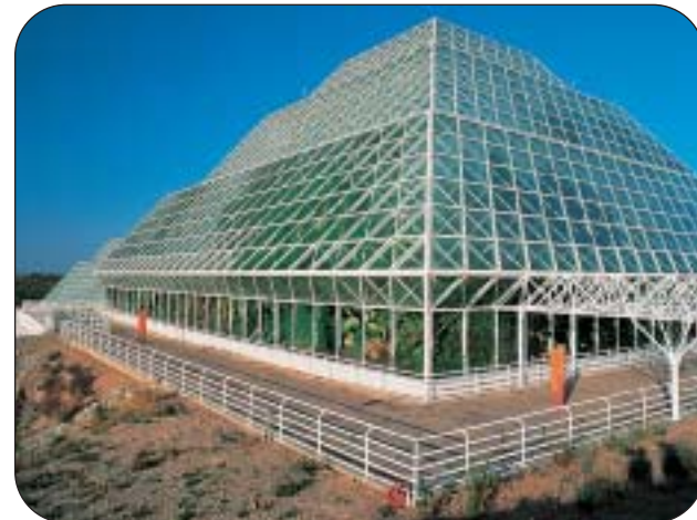
Science under glass. Columbia University’s Biosphere 2, a huge glass and metal ecological research facility located 20 miles north of Tucson, Ariz., is a three-acre test tube meant to mimic Biosphere 1—planet earth. In this kind of model, would decision makers’ rationality be less bounded?
