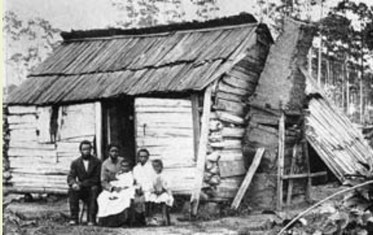
Chimneys on sharecroppers' cabins were often tilted deliberately so that they could be pushed away from the house quickly if they caught fire.
