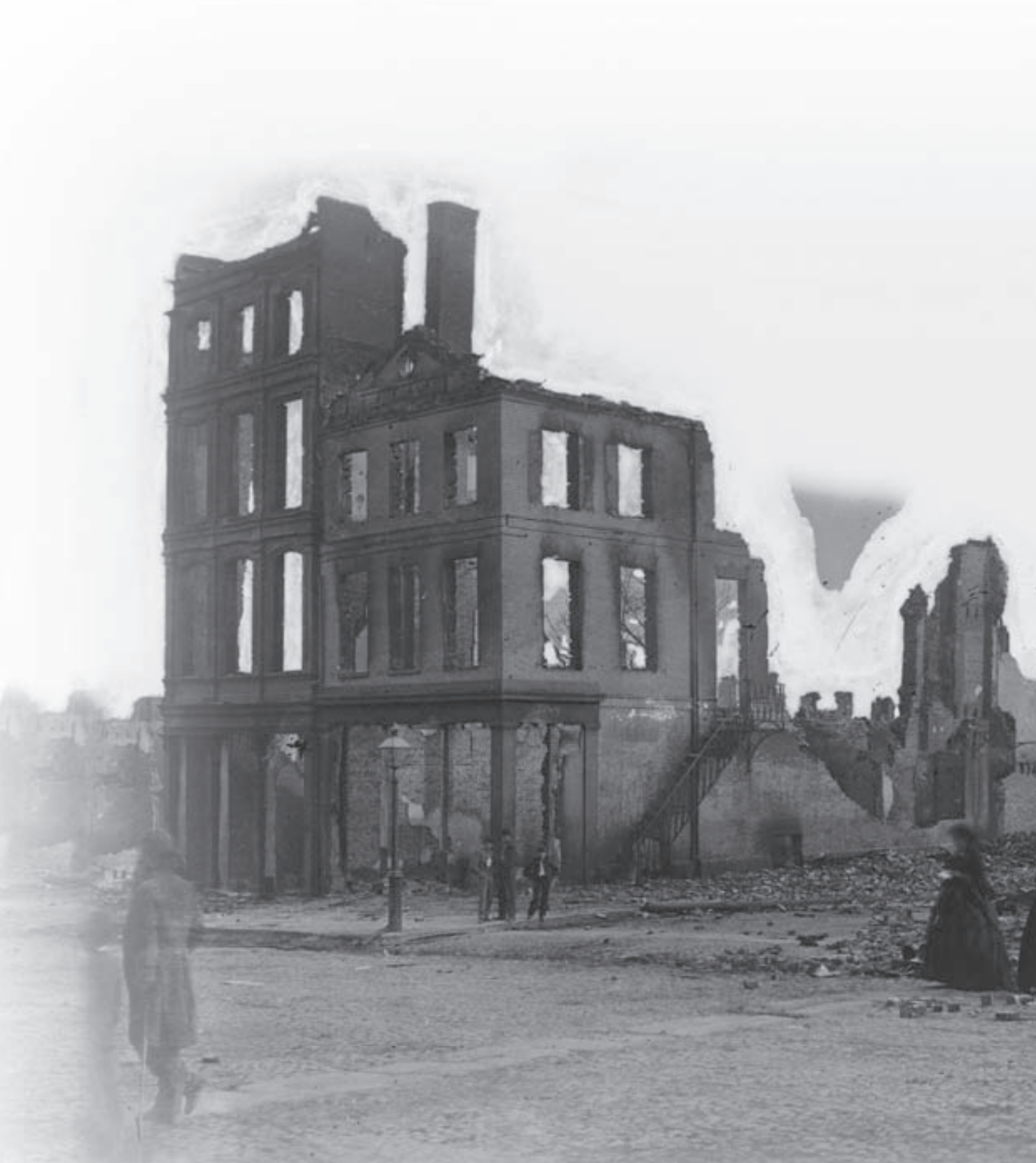
“There were swaying chimneys, tottering walls, streets impassable from piles of brick, stones, and rubbish,” reported one journalist in Richmond at war’s end. “Men stood speechless, haggard . . . gazing at the desolation.” In this photograph, the need for a time exposure made residents walking the streets look like ghosts. Many must have felt that way in defeat, though newly freed African Americans were exultant.
