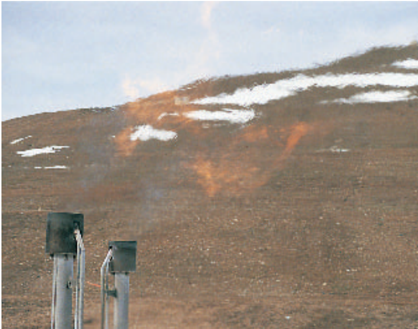
Figure 13 Methane gas produced by bacteria in this landfill is burning at the top of these collection tubes.
